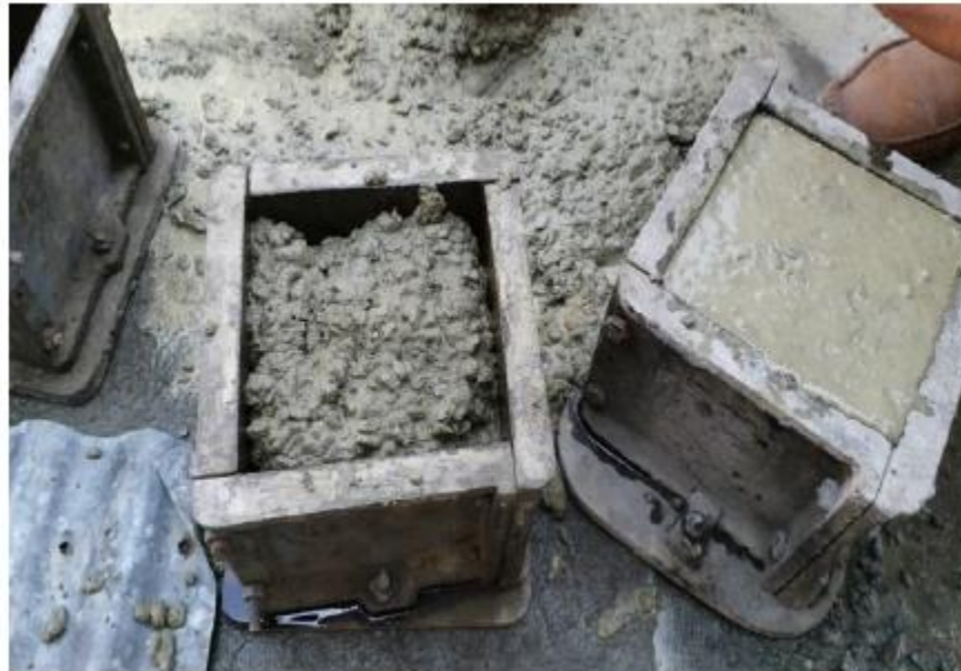
Fig. 3: casting of 150mm concrete cubes.
